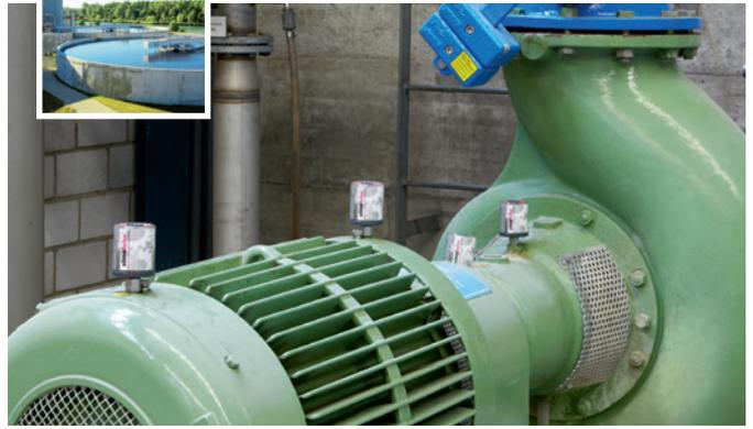
60 ml lubricators on the electric motor and the drive shaft ensure continuous lubrication of a centrifugal pump.
