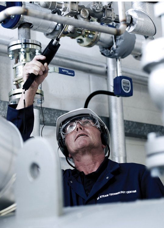
An Engineer carrying out steam system audit
