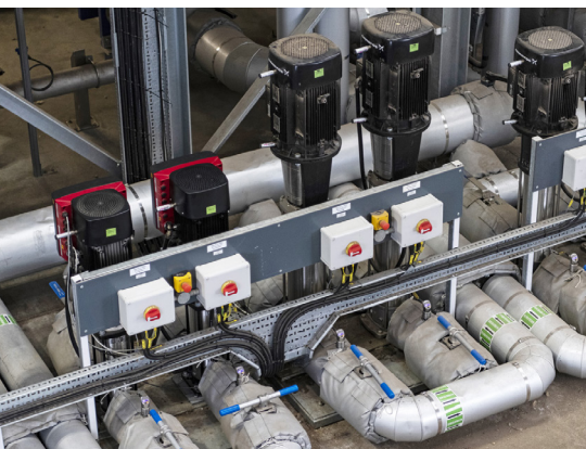
Grundfos CRIE pumps have built-in variable speed drives. These replace the usual modulating valves
