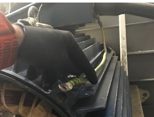
Remedial engineering work on NDE drive motor
