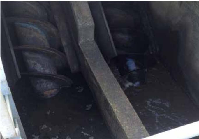
guide. Cutting equipment then removed a given section of flight to return the flights to a parallel consistency along its entire length.
